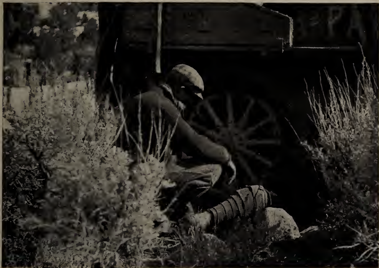
ROCKY MOUNTAINS: REPAIRS IN THE JUNGLE.
